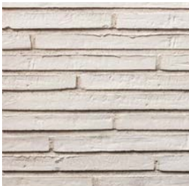
(Br2) WHITE BRICK RECESSED JOINTS
