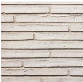
(Br2) WHITE BRICK RECESSED JOINTS
